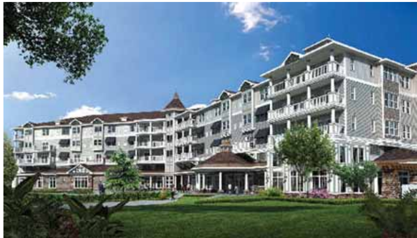
Watkins Glen Harbor Hotel, currently under construction on the Seneca lakefront.
